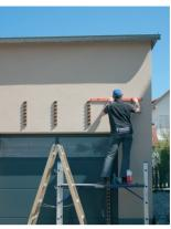
Install battens vertically and levelled in horizontal direction.
